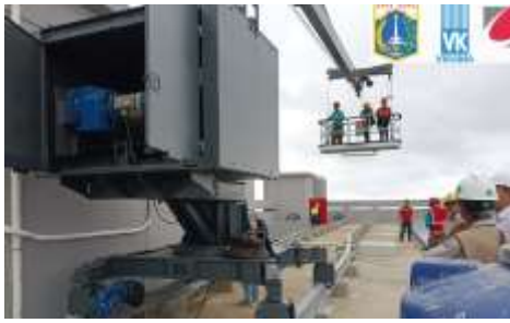
Gambar 9. instalasi lengkap Gondola (Building Maintenance Unit / BMU)
