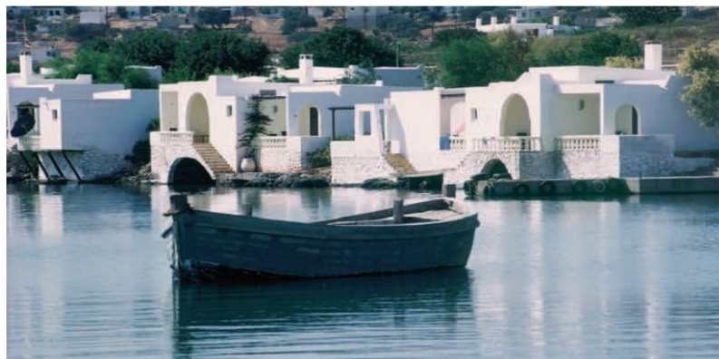
Figure 2. Tourist accommodation in Corfu, Greece, with forms designed to accord with concepts of the vernacular architecture of the island (Source: Paul Oliver's 'Built to meet needs')
